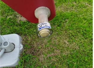
The ends of the footrests have a cross section of less than 15cm2 and fail to meet the requirements of BS EN 1176 Finding:
