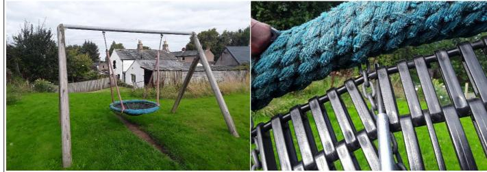
**Finding:** The openings between the slots in the Basket Seat **Action:** Monitor Use
